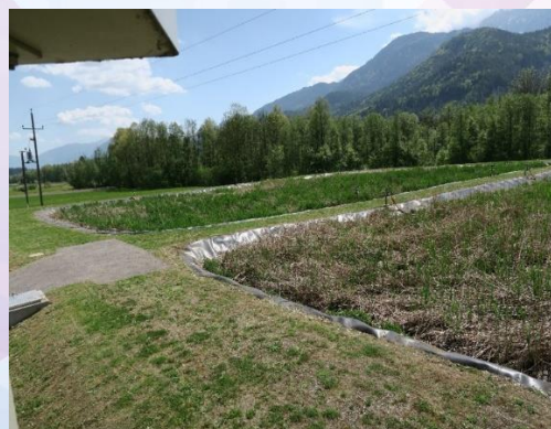
Sludge drying reed bed scheme (left) and live (right) (source: Limnos)
